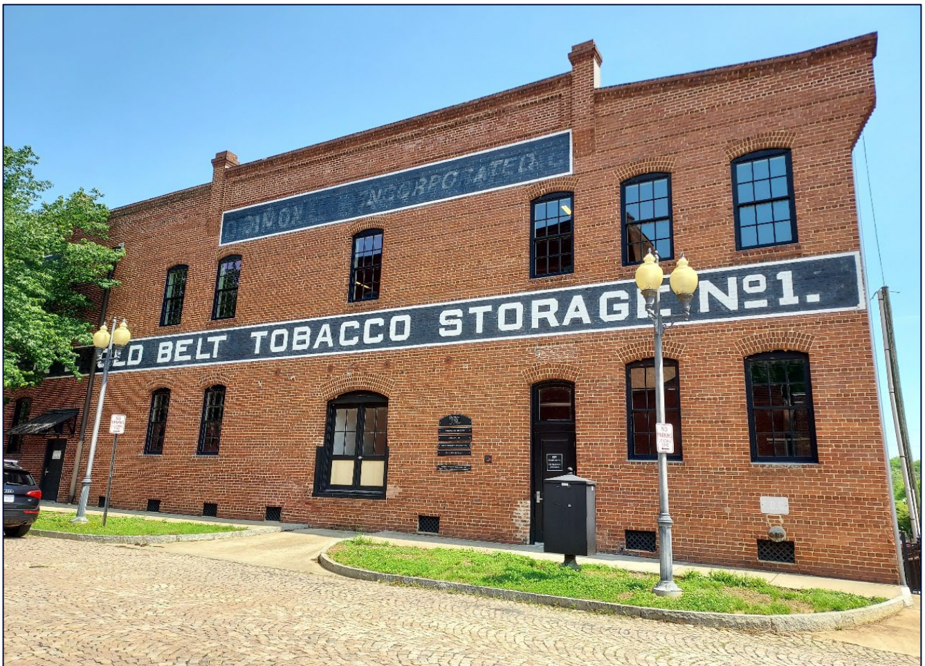
Figure 1-2: Old Belt Tobacco Storage Building
