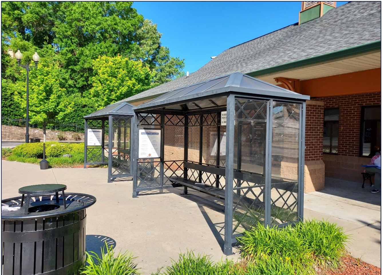
Figure 1-8: Danville Transit Bus Shelters at the HUB
