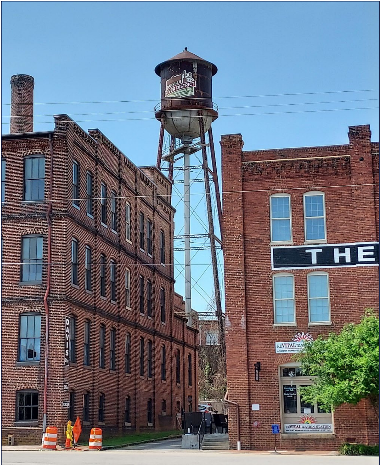
Figure 1-3: Danville River District Buildings Under Renovation
